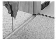
In doorways, mount a suitable moulding system to ensure the necessary expansion space. This also applies if the same floor is to be laid in the adjoining room. In this case, a transition moulding should be used for covering the required expansion gap.
