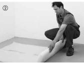
Always use 0.2 mm thick PE film overlapped by 30 cm as an underlay when laying your floor over floor screed. This should overlap in the 30 cm impact area. Extend underlay up all walls. After having installed the skirtings cut underlay at the upper edge of the skirtings.
