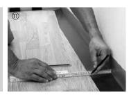
Cut to size and fit in the boards of the last row. Leave a gap of 10 to 15 mm between the boards and wall.
