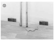
If radiator pipes protrude from the floor, drill or saw a cutout into the board (the size of the cutout depends on the radiator pipe and the required expansion space).
