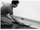
The next row is started with the leftover piece of the first row (short side offset of at least 50 cm). This considerably reduces waste. The rest of the installation is performed boardby-board. First, the boards are angled into the previous row along the long side by applying a small amount of force.
