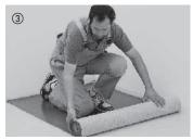
For sound insulation and to smooth out slight irregularities of the subfloor, unroll 2 mm thick luxury insulation layer. Our range of accessories also offers suitable insulation underlays. Asphalt-bitumen felt is not suitable for sound insulation. Parquet with integrated insulation layer is not suitable for glue-down installation.
