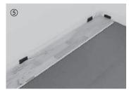
Starting in the right-hand corner of the room, align the boards of the first row with the tongue side parallel to the wall, and fix them in place with wall spacers or plastic spacers as you proceed (always keep an expansion gap of 10 - 15 mm (3/8 " – 1/2") around perimeter).
