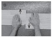
Unlocking of Top Connect: The boards can be pushed out from one another parallel.
