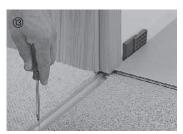
In doorways, mount a suitable moulding system to ensure the necessary expansion space. This also applies if the same floor is to be laid in the adjoining room. In this case, a transition moulding should be used for covering the required expansion gap. Leave an expansion space of approx. 5 mm between the board and the base of the moulding. As a rule, a fine saw must be used to cut a gap the thickness of a board in wooden door frames to allow the parquet to expand.
