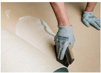
For the installation of linoleum floors use suitable dispersion adhesives, for example 611 Eurostar Lino (Forbo Eurocol ) or equivalent. After application of the adhesive (with a notched trowel TKB-B1), the sheets are pushed or rolled into the wet adhesive bed, observing the laying time into the wet adhesive bed. Any adhesive stains can be removed immediately with water (Attention: Do not use nitro thinners, products containing solvents or aggressive cleaners).
